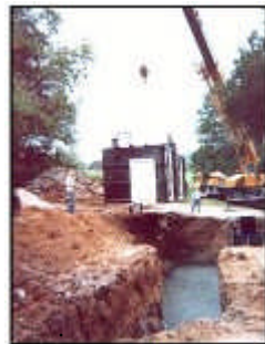
Shelter being lowered into wet cement.
