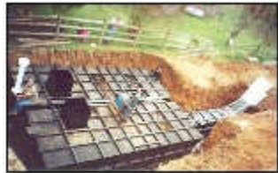
Two 7' x 8' x 25' shelters with 20' long walkway and blast door.
